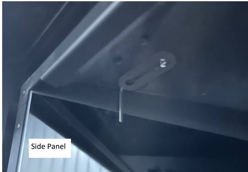
Figure 6 - Side Panel Clip Installation
