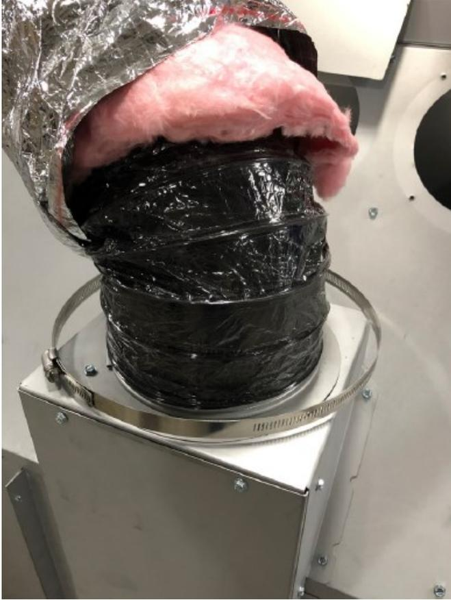
Figure 2.3, Attach Inner duct
