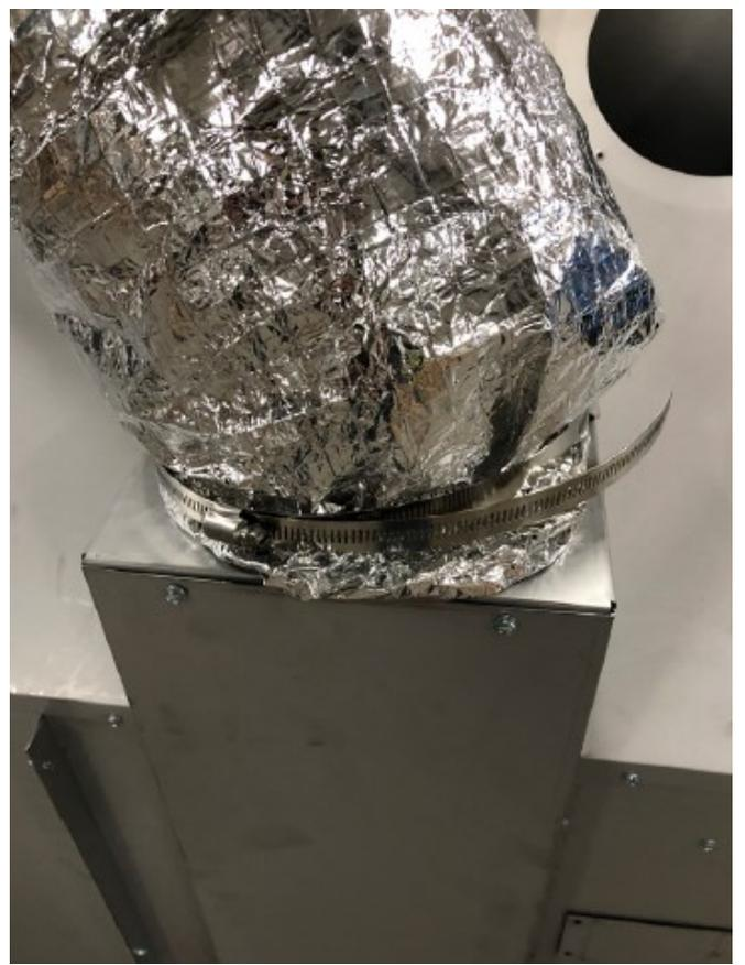
Figure 2.4, Band clamp securing insulation
