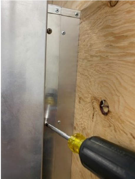
Figure 4.1 - Remove Cover Assembly
