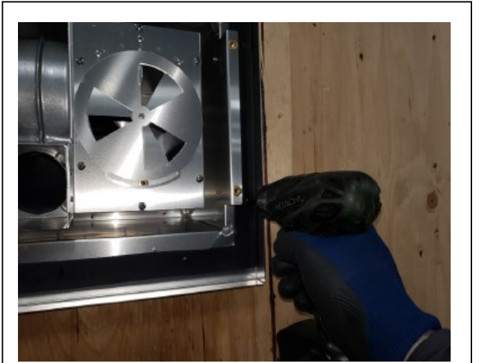
Figure 6.6 - Secure Power Vent to Exterior
