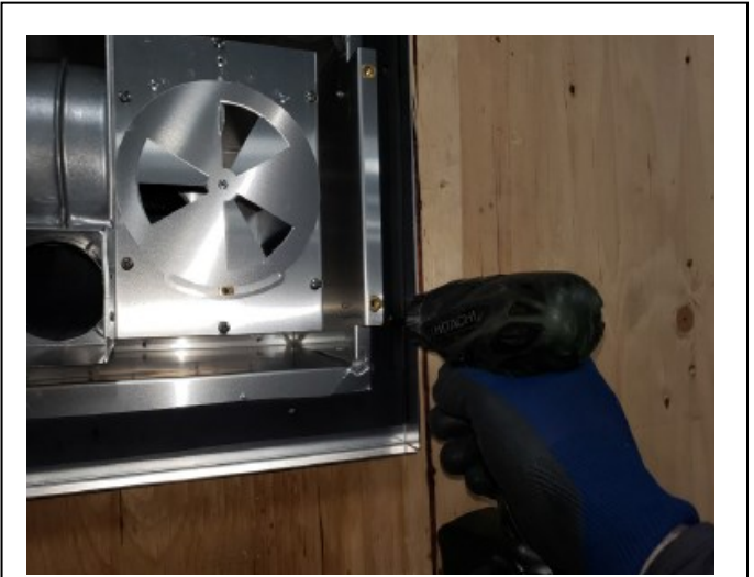
Figure 6.6 - Secure Power Vent to Exterior
