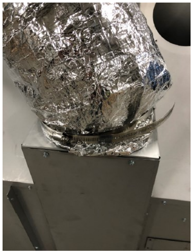
Figure 2.4, Band clamp securing insulation
