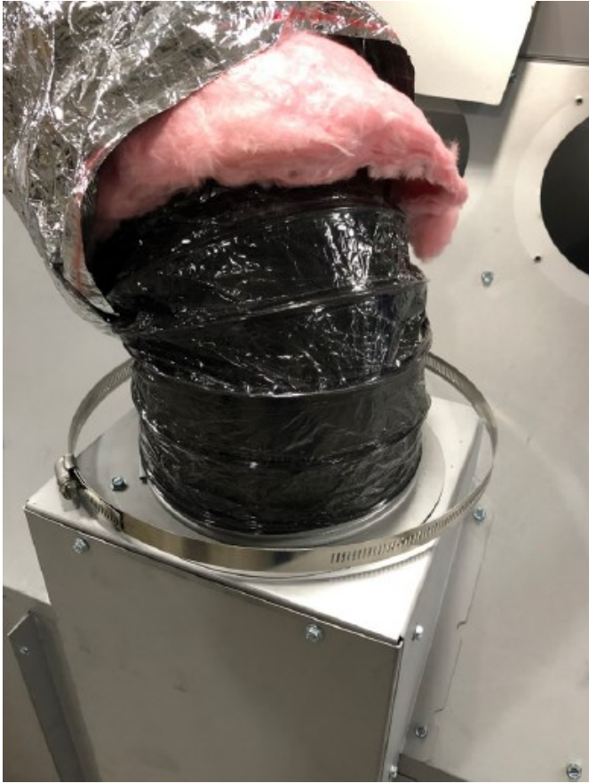
Figure 2.3, Attach Inner duct
