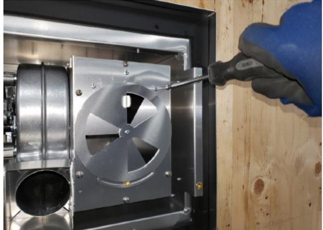
Figure 8.2 - Exhaust Assembly Screws
