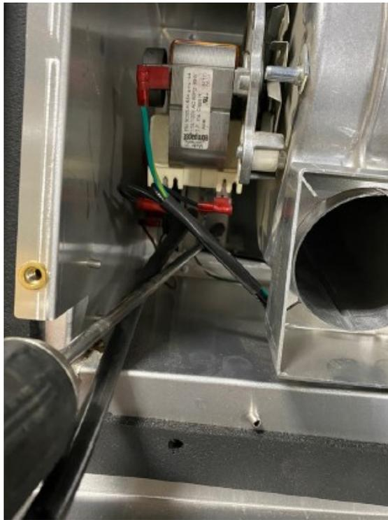
Figure 8.9 - Vacuum Switch Removal
