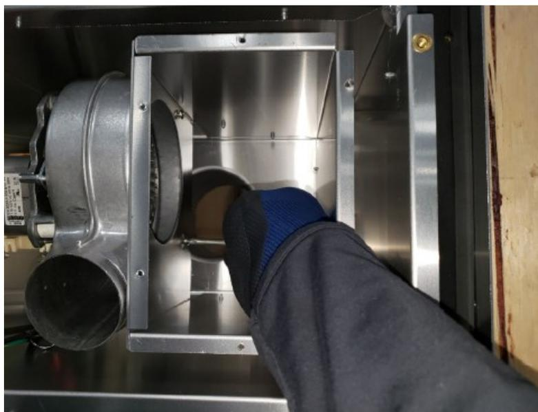
Figure 8.6 - Remove (3) Screws Securing Fan Assembly
