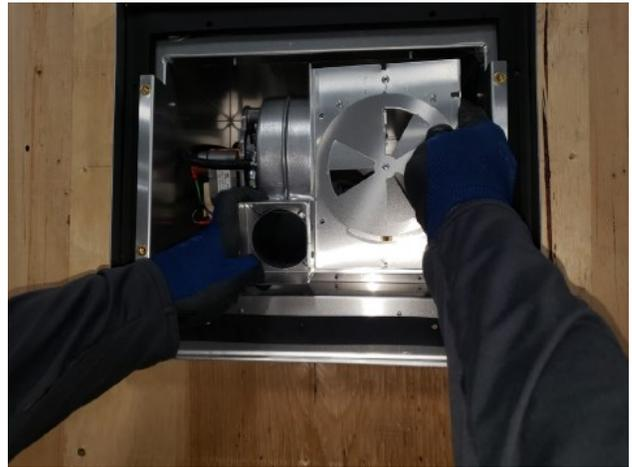
Figure 8.3 - Exhaust Assembly Removal
