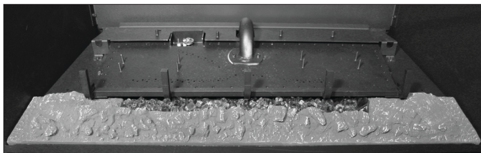
Figure 9.3, Completed Light Kit Installation
