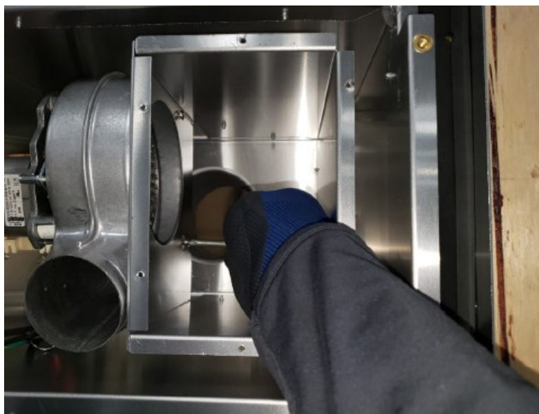
Figure 8.6 - Remove (3) Screws Securing Fan Assembly
